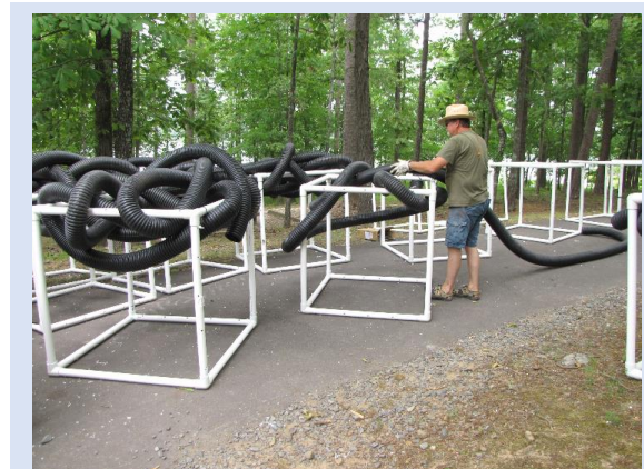
"Georgia Cubes" made from PVC and corrugated drain pipe.
